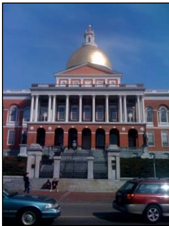
Capitol Building in Boston. Part of the Freedom Trail walking tour.
